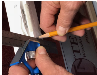
Mark position of new lock over notches of old lock.
