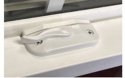
Permanently fasten new lock in same position as old lock.
