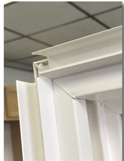
Drywall Return Available for 1/2" and 5/8" drywall.
